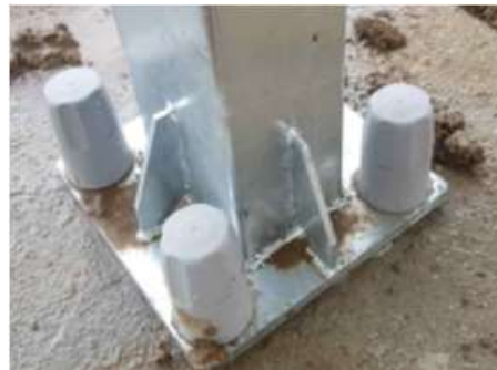
Column Rod Welding
